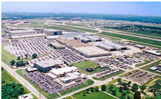
The sprawling Tulsa maintenance base covers more than 300 acres of land.
